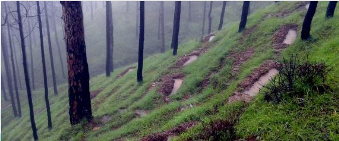
A series of trenches/ Khantis along hill slopes hold rainwater and recharge water sources, Uttarakhand
